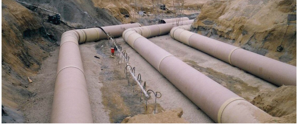
GRP pipe for desalination plant. (Picture courtesy of Amiantit.)
