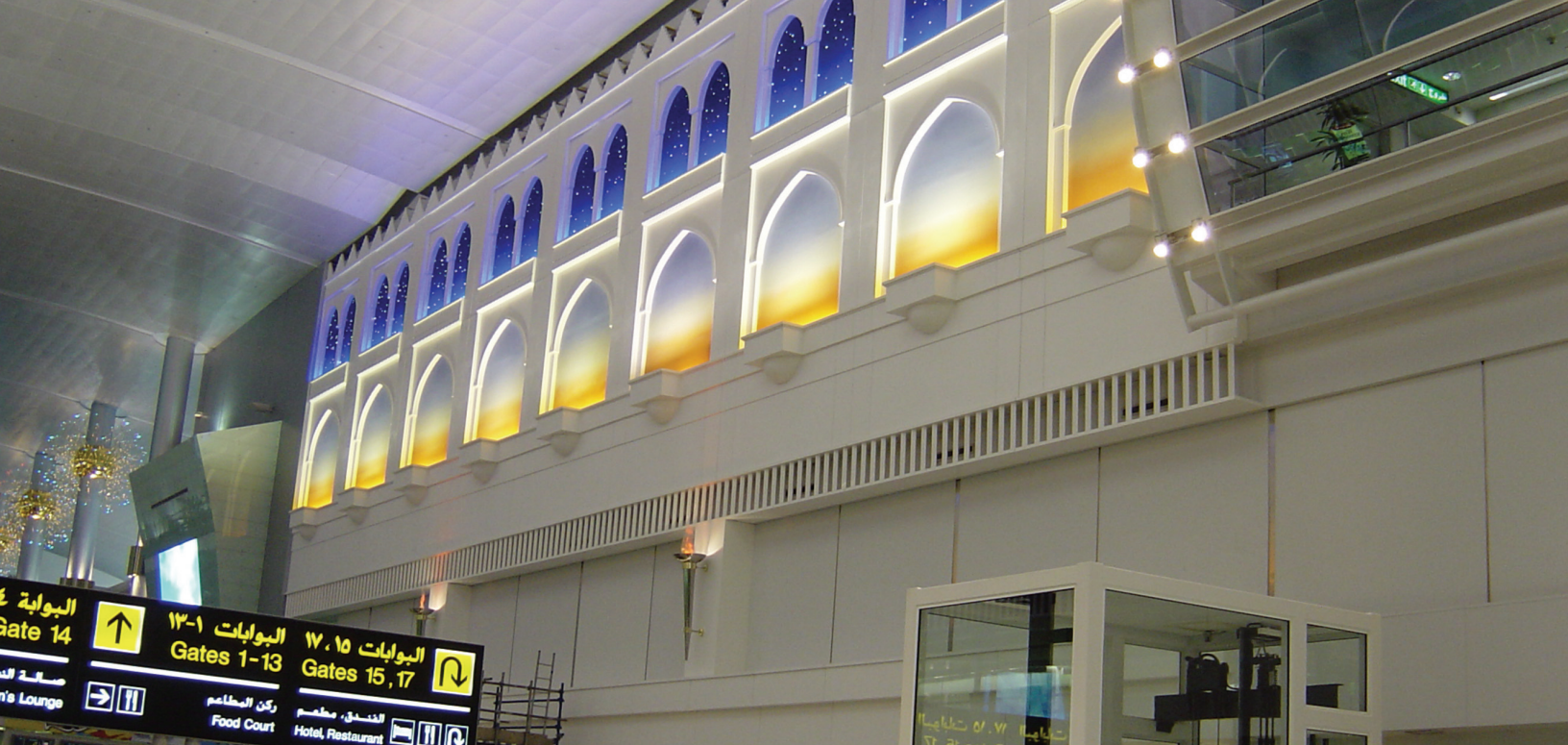
GRP cladding at Dubai International Airport. (Picture courtesy of Terrazzo Ltd.)
