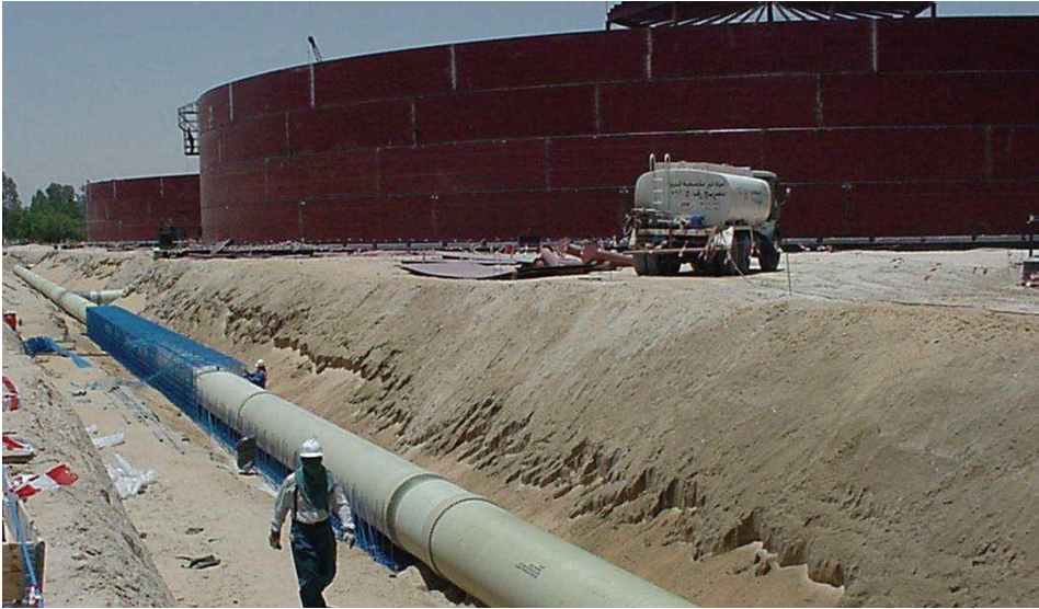
GRP sewer pipe. (Picture courtesy of Amiantit.)
